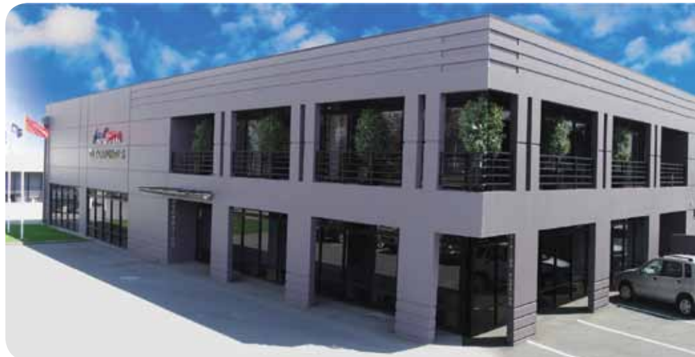
AuCom manufacturing plant in Christchurch, New Zealand.
